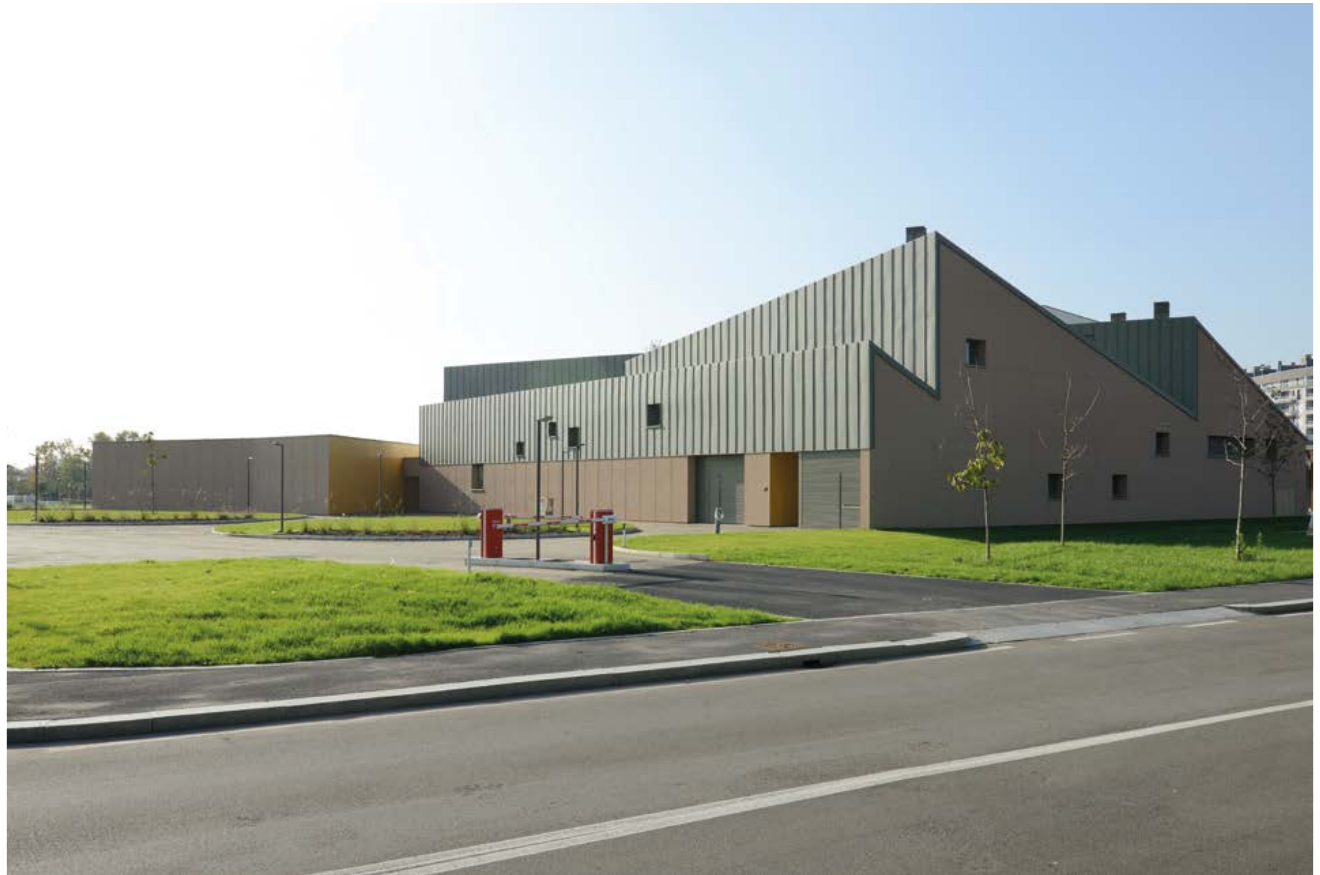
↑ Multi-purpose building for demonstrations and events / ph Michele Nastasi / © Calzoni Architetti | Sonia Calzoni
